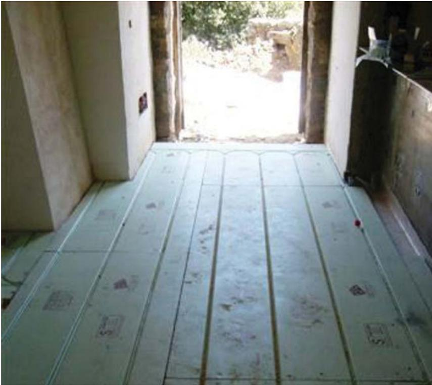
Radiant floor heating and cooling is distributed throughout the home with PEX tubing in a grooved subfloor. The radiant cooling system draws water from the rainwater collection cistern.
